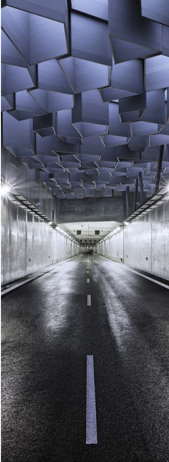
Nordhavn Tunnel Denmark
