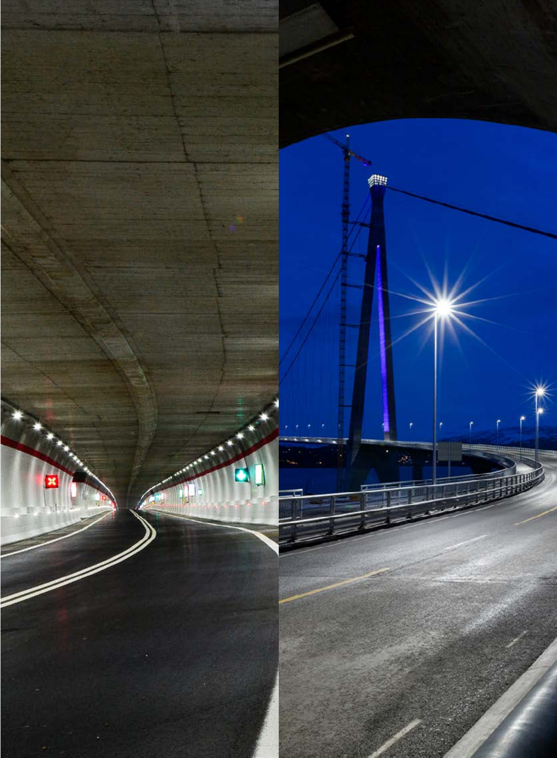
Valnerina Tunnel Italy
